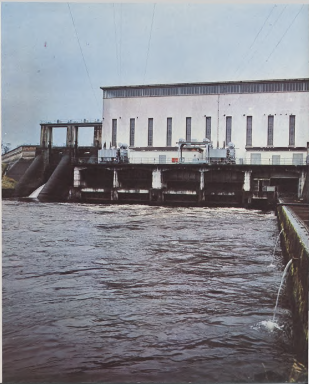
Cliff Generating Station
