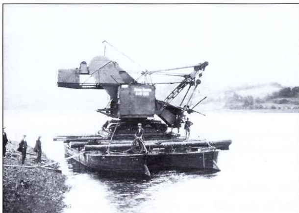
■ Transport of bucket excavator on two barges. Source: Siemens Progress on the Shannon, Number 11, August 1927.
