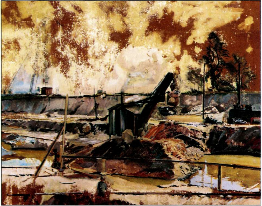
■ Commencement of tailrace. Excavation work for canal and building of banks.
