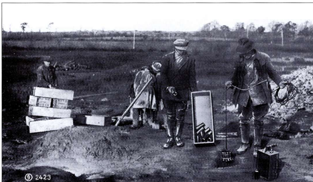
■ Charging the bore holes.
