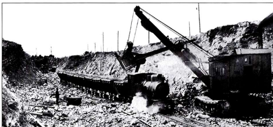
■ Bucket excavator and train in action. Source: ESB Archives Photographic Collection.
