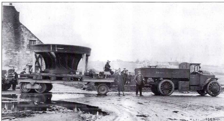
■ Transporting the runner of one of the Francis turbines from Longpavement, 1928.
