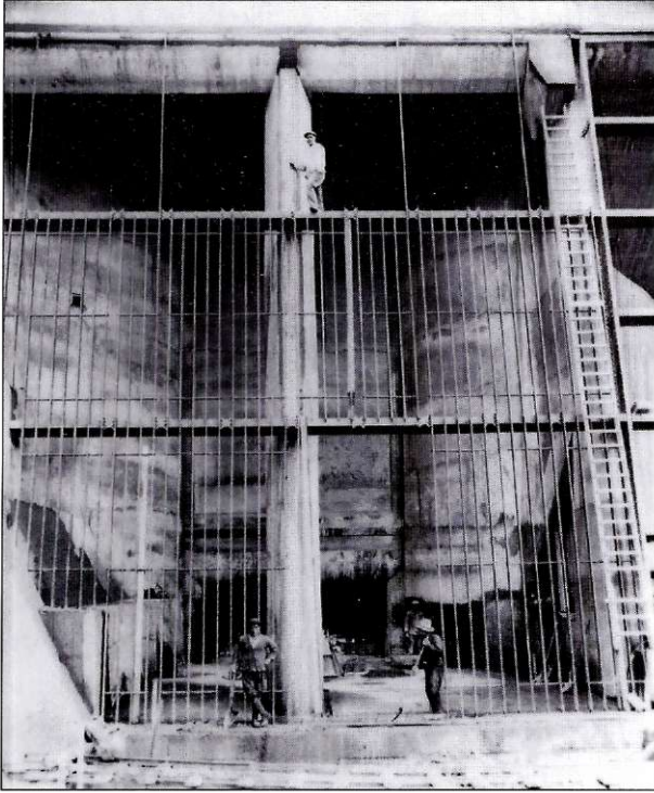
■ Concrete work for power house. Source: ESB Archives Photographic Collection.
