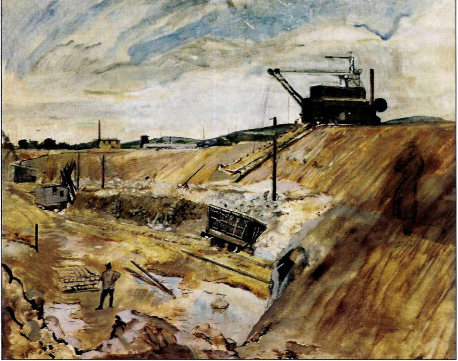
■ Excavator at work, Lubecker with stone wagon and steam shovel.
