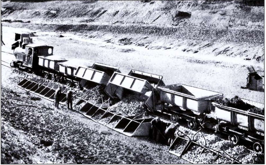
■ Conveying broken stones.
