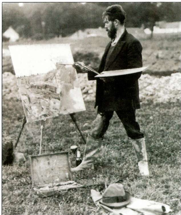
■ Sean Keating on site at Ardnacrusha 1927. Source: The Cashman Collection .
