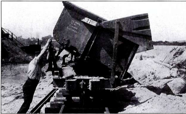
■ Krupp tipping-wagon. Source: Siemens, Progress on the Shannon, Number 6, March 1927.
